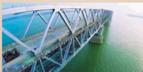
Greenfield Bridge in Ganga Near Bakhtiarpur
